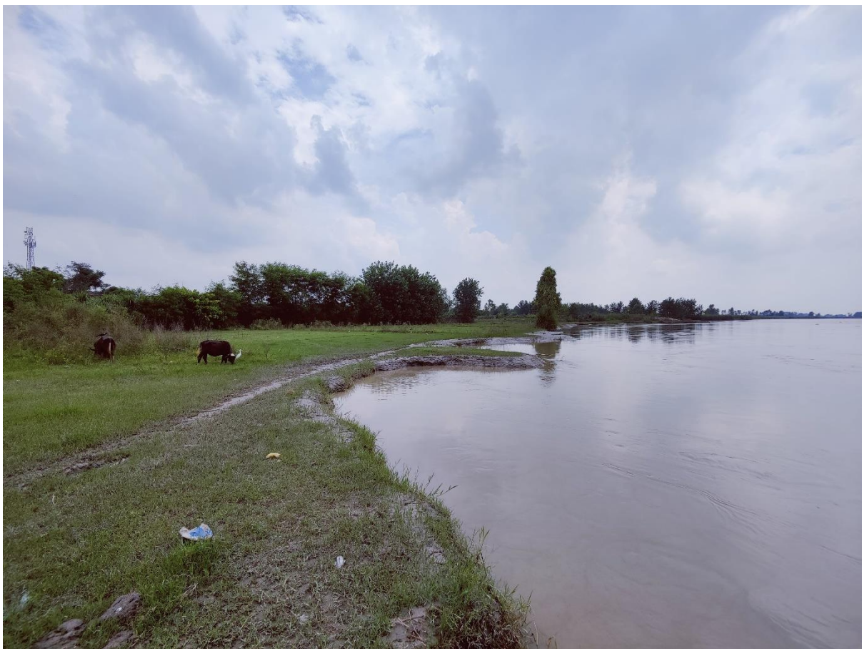
Image 28 : River Bank Erosion At Chaupura Khadar, Distt. Amroha
