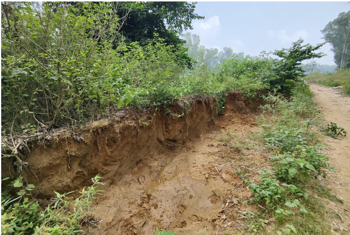
Image 33 : Mined River Embankment Area Near Bhojpura
